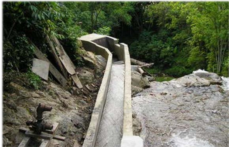
Figure 5: Existing Hydrological Structure
